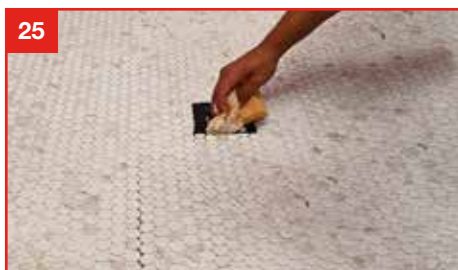
25. Remove the protective cover and clean the excess thinset and replace the cover.
