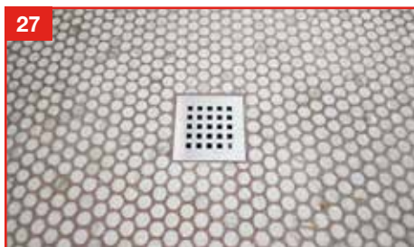
27. Finally, remove the drain cover and place the chosen grate.
