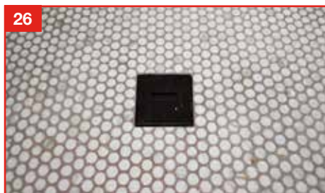
26. With the protective cover in place, grout the entire floor.
