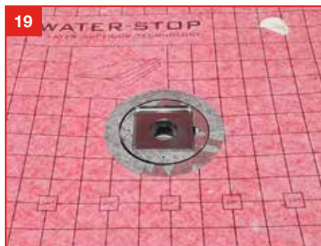
2. Place the drain on the drain housing.
