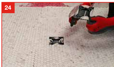
24. Repeat the process with the grate holder, applying thinset and installing the piece onto the spacers.
